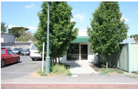
26A Aitken Street GISBORNE VIC
